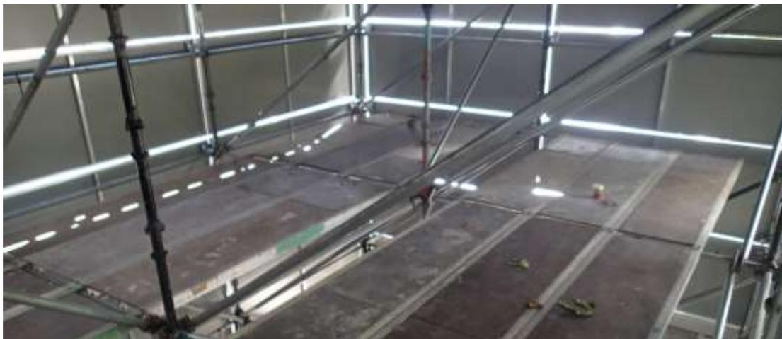
*SEWPS decks within a scaffold tower (with external cladding in place)*
